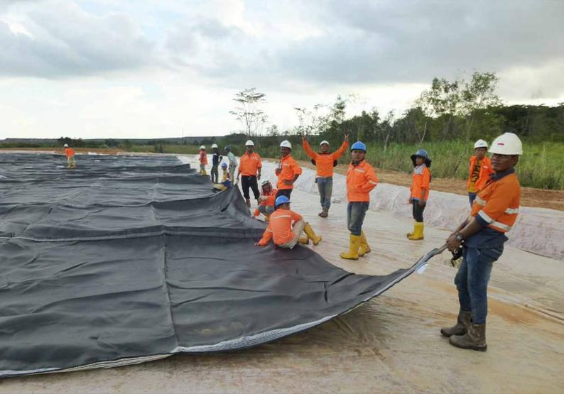
The Geotube<sup>®</sup> dewatering unit was positioned on the drainage platform according to the layout plan.
