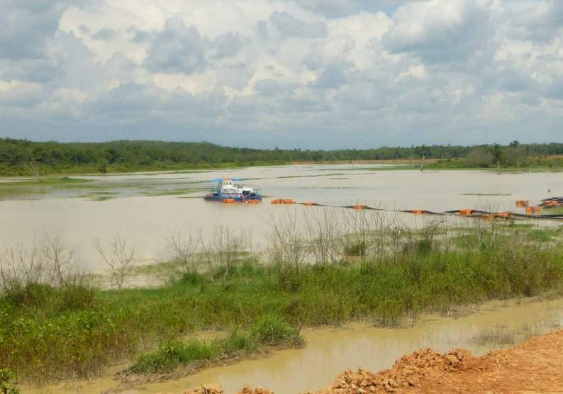
A dredger was deployed to transfer silt sediment slurry to the dewatering platform. The dredger had a pumping flow rate capacity of 400 to 550m<sup>3</sup>/hour.
