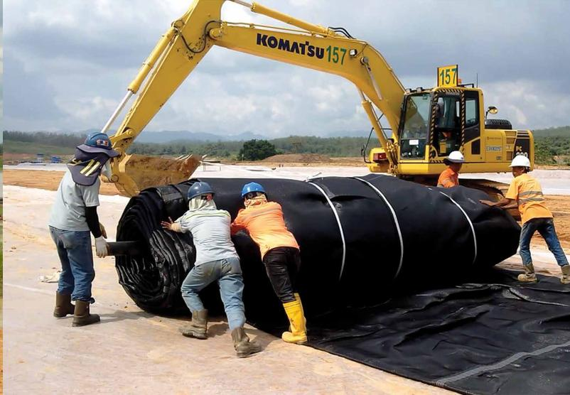
An excavator was used to assist in rolling out the Geotube<sup>®</sup> dewatering unit into position on the dewatering platform.
