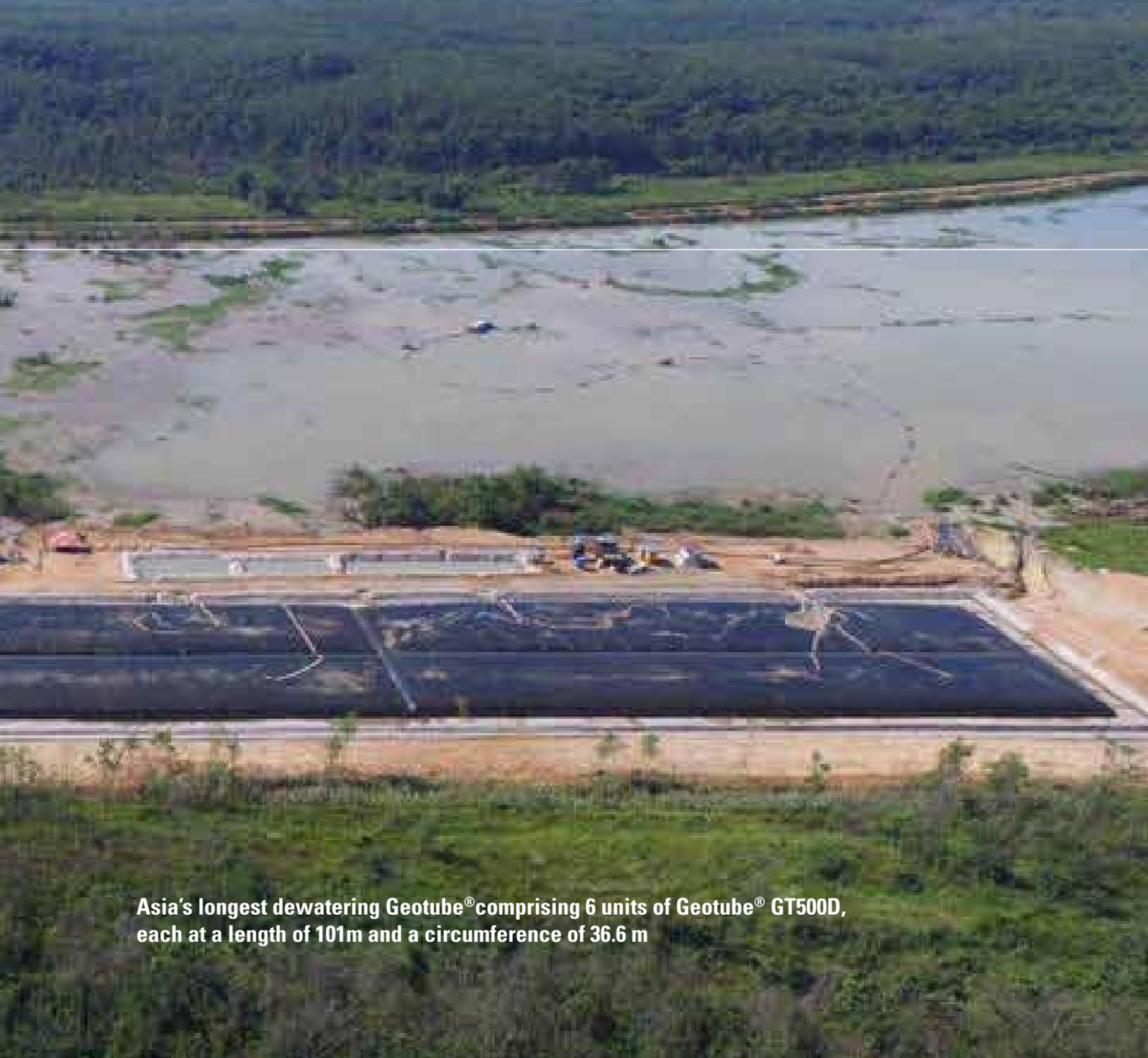
**Asia's longest dewatering Geotube® comprising 6 units of Geotube® GT500D, each at a length of 101m and a circumference of 36.6 m**
