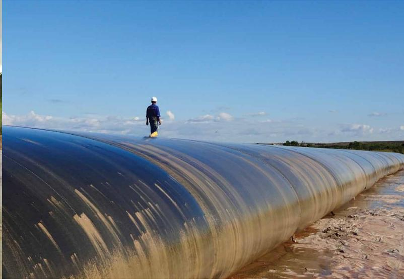
The Geotube<sup>®</sup> dewatering unit was filled to the maximum controlled height.
