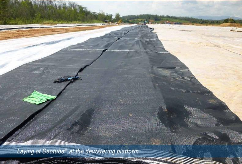
Laying of Geotube® at the dewatering platform
